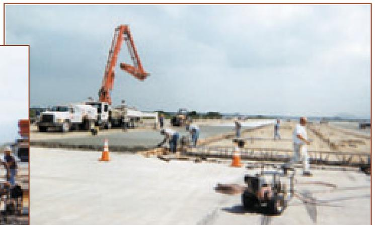
Point Mugu Naval Air Station required a 565 foot long non-jointed pour of 30% Class F fly ash concrete.
