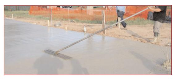
Finishing the 75% fly ash concrete was done with ease, despite initial concerns that finishing would be more difficult compared to conventional concrete.
